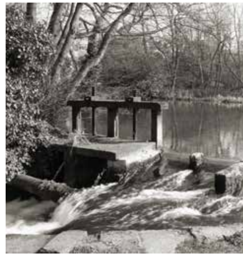
Arundel Mill Pond Sluice Gate
