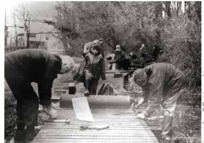
Installing boardwalk at Frome Banks
