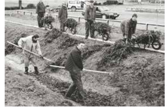
Reed transplanting work at Stratford Park
